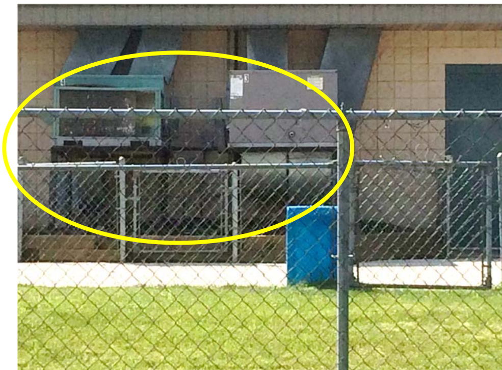
View from Erickson Way on the east side of the facility
