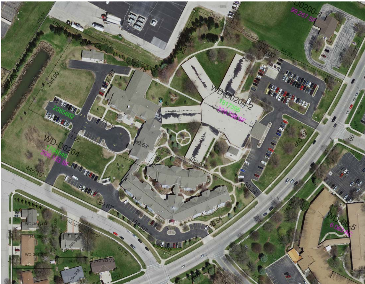
Figure 1. Image of existing site.
