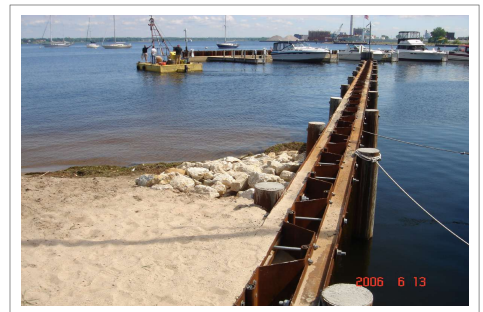
Harbor North SSP Breakwater
