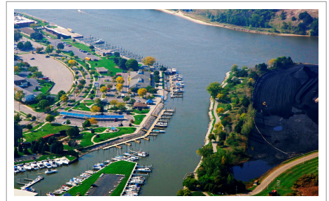
Aerial View of Fixed and Floating Docks
