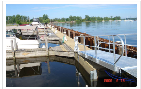
South SSP Breakwater and Floating Docks
