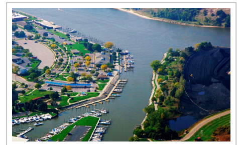
Aerial View of Fixed and Floating Docks
