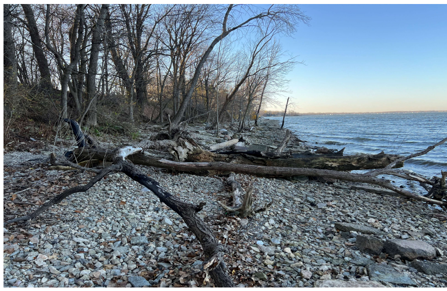
Shoreline Erosion and Storm Damages
