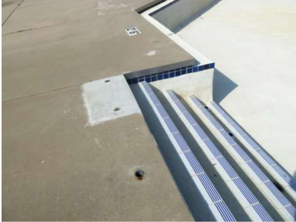
Handrail Anchors for New Stair ADA Access
