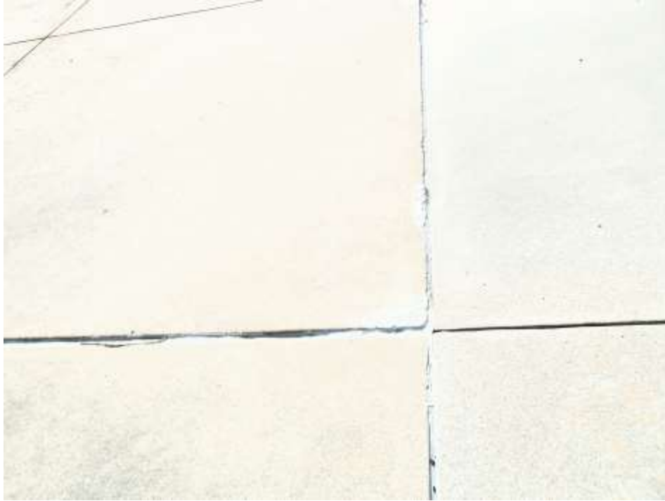
Pool Deck Joints Require Repair
