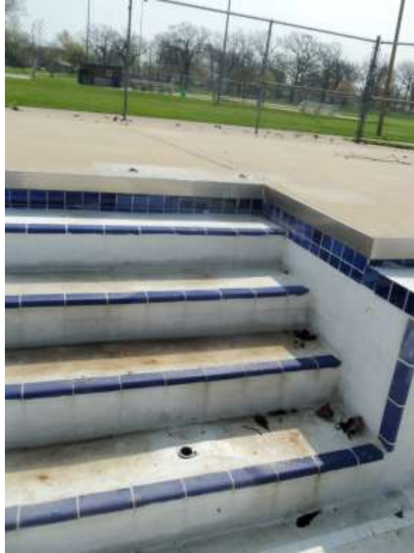
Pool Stair was repaired. Concrete was deteriorated
