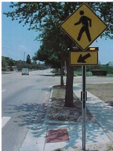
Figure 10: Pedestrian Crossing Rectangular Rapid Flashing Beacon (RRFB)
