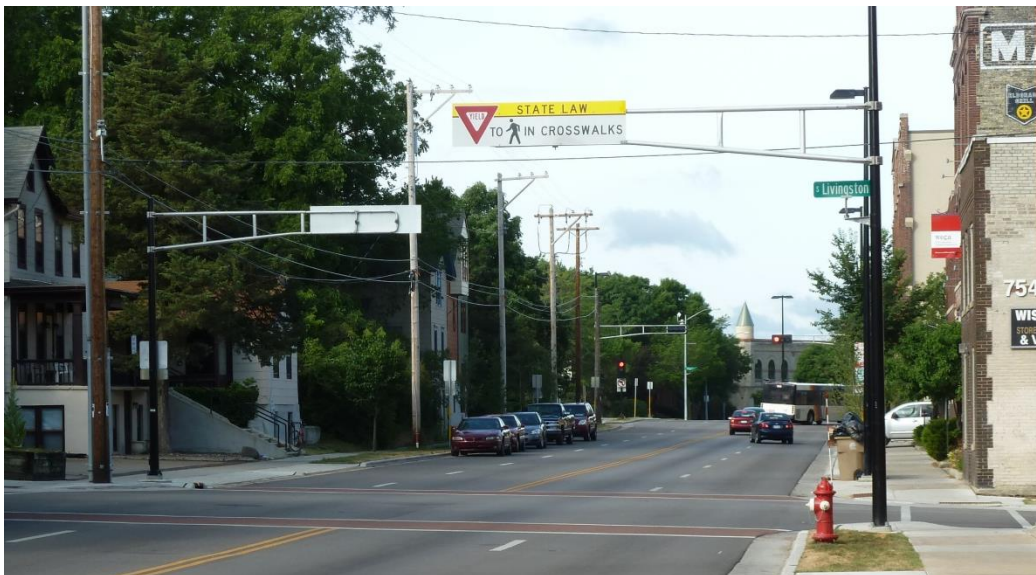
Figure 9: Overhead ‘Yield to Pedestrians in Crosswalk’ Sign
