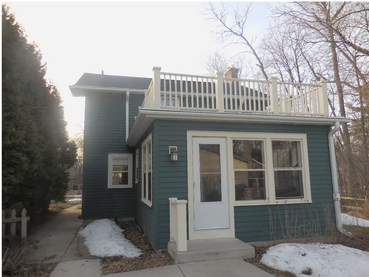
933 Oakdale Avenue Back Porch added in 2012 It does not cancel the History Character of the house because it is not visible from the street front facade.
