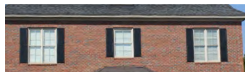
Inappropriately Scaled Shutters: Not Permitted
