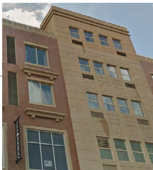
Figure 9-13. Utility Appurtenances located on Facades
