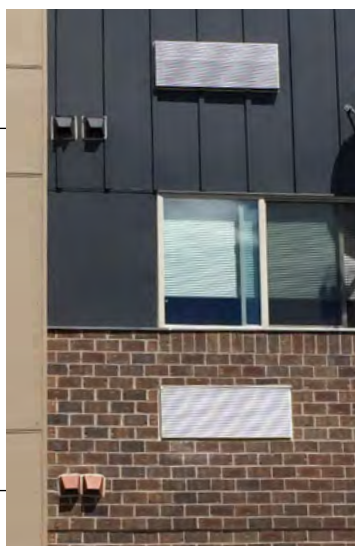
Figure 9-13. Utility Appurtenances located on Facades
