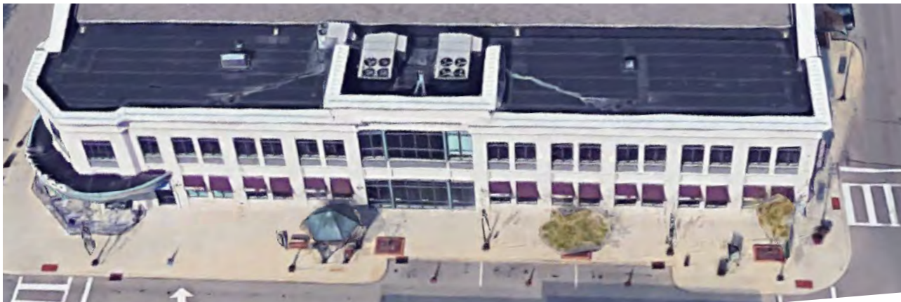
Figure 9-12. Rooftop Utilities Screened from the Public Way by a Parapet
