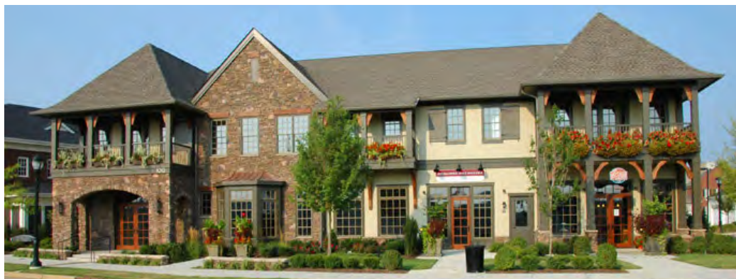
Figure 3-5. Illustrative Examples of Commercial Manor Building
