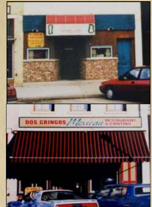
Recommended window replacement
