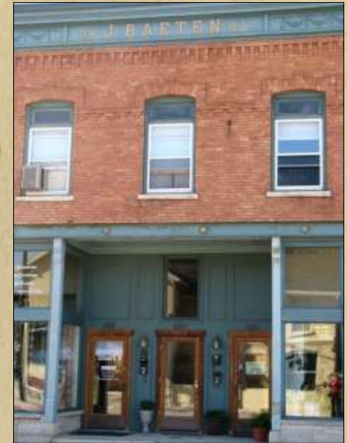
Recommended preservation of building's metal.
