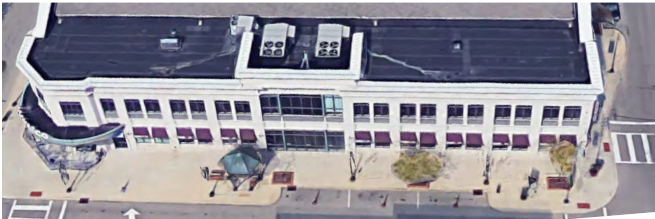
Figure 9-11. Rooftop Utilities Screened from the Public Way by a Parapet
