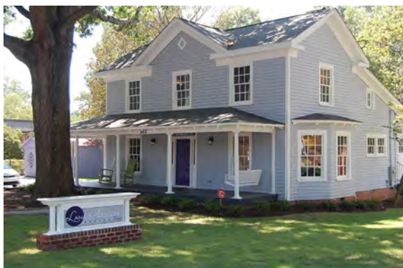
Figure 3-5. Illustrative Examples of Commercial Manor Building
