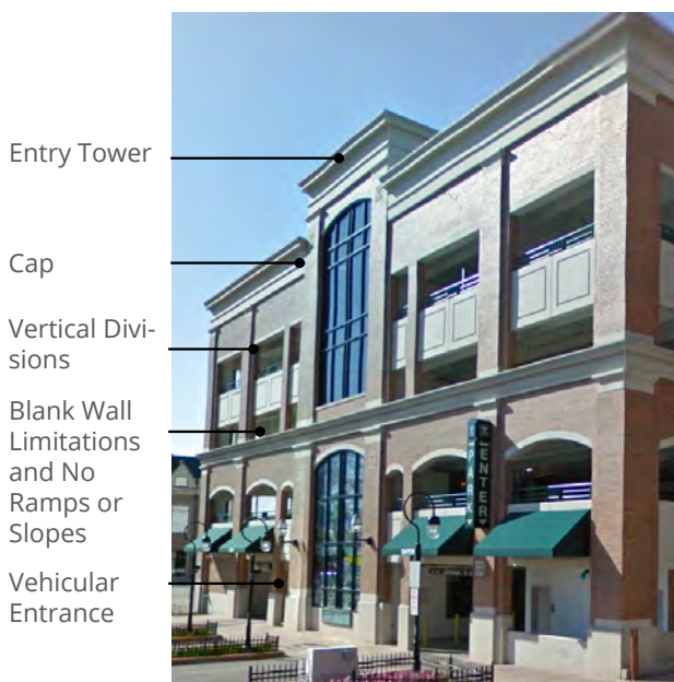
Figure 9-14. Illustration of Parking Structure
