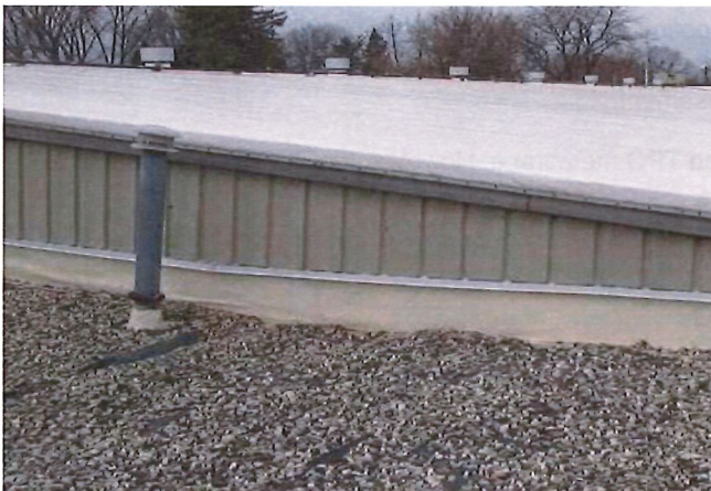
ARENA AND ICE PLANT ROOF
