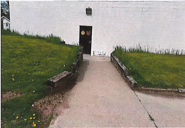
WOODEN RETAINER WALLS
