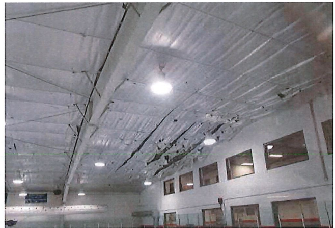
REFLECTIVE MEMBRANE RIPPED BY PUCKS
