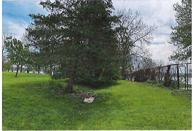
EAST DRAINAGE SWALE
