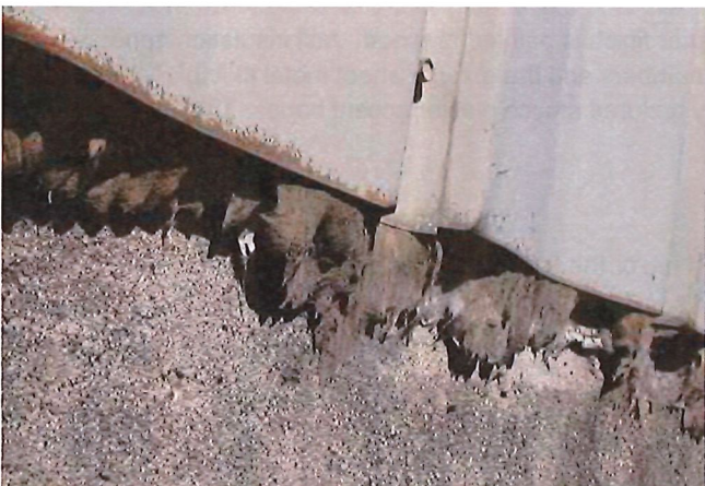
EXPOSED WALL INSULATION AT WALL BASE
