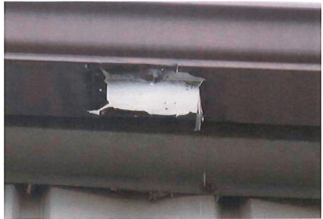
MISSING DOWNSPOUT
