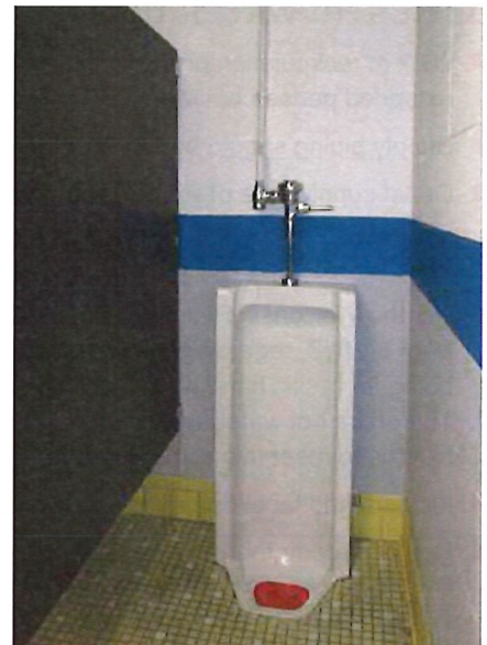
2ND LEVEL STALL URINAL MANUAL FLUSH
