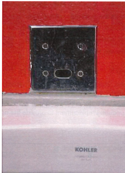
URINAL SENSOR OPERATED FLUSH
