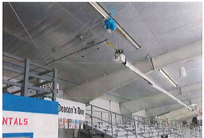
INFRARED HEATERS
