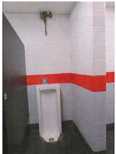
STALL TYPE URINALS W/SENSOR OPERATED FLUSH
