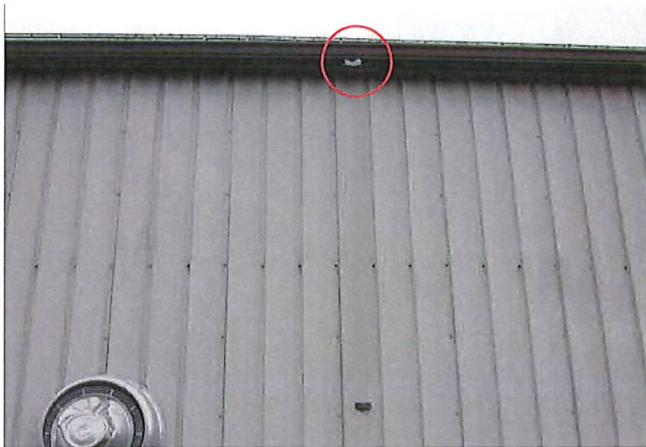
MISSING DOWNSPOUT
