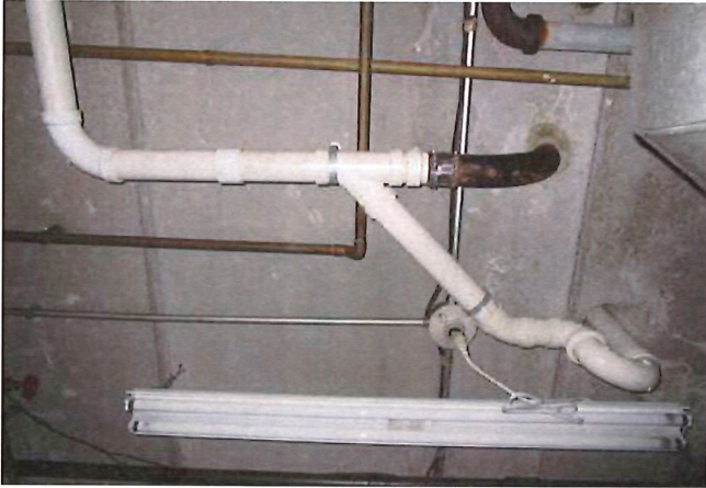
REPAIRS IN PVC
