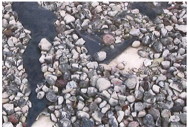
ICE PLANT ROOF
