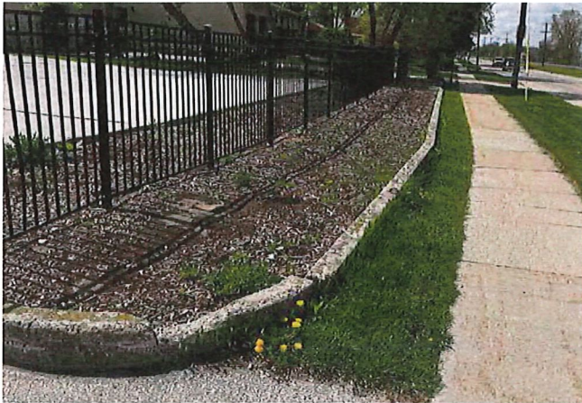
RETAINING CURB AT FORT HOWARD DRIVE
