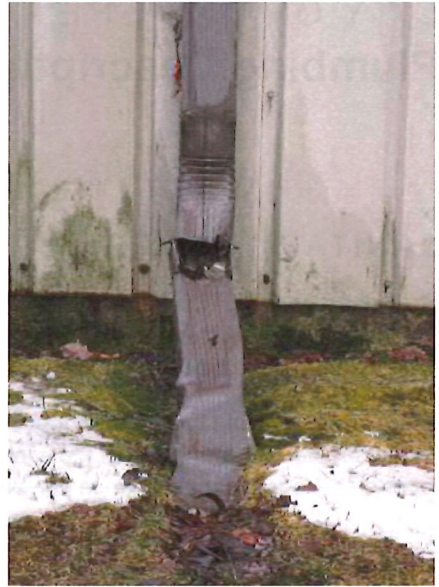
CRUSHED DOWNSPOUTS
