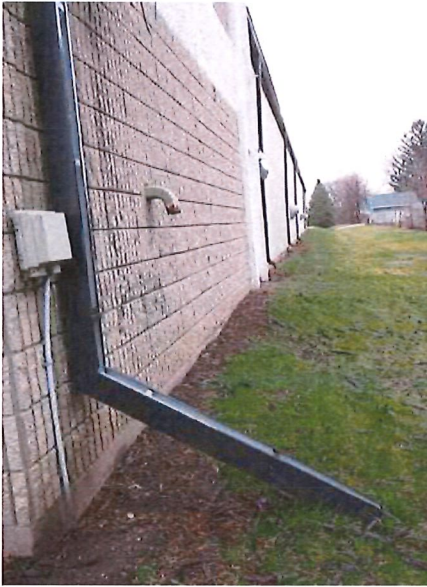
GUTTER AND DOWNSPOUTS
