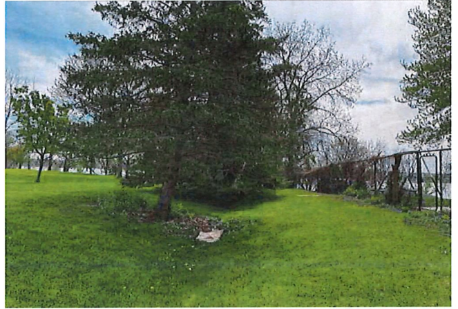
EAST DRAINAGE SWALE
