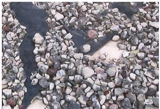
ICE PLANT ROOF
