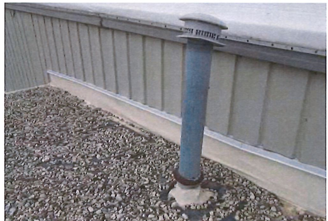
UNIT HEATER FLUE VENT
