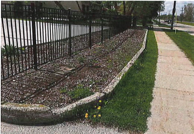
RETAINING CURB AT FORT HOWARD DRIVE
