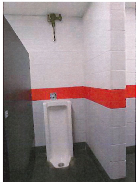
STALL TYPE URINALS W/SENSOR OPERATED FLUSH
