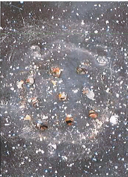
SHOWER ROOM FLOOR DRAIN GRATE
