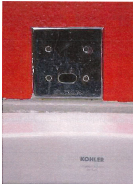
URINAL SENSOR OPERATED FLUSH
