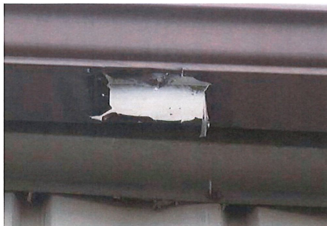
MISSING DOWNSPOUT
