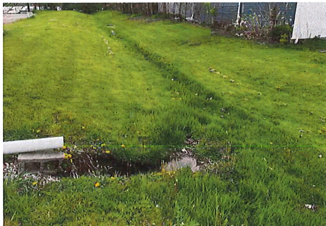
SOUTH DRAINAGE SWOLE
