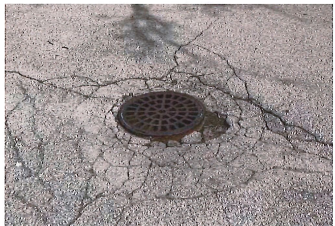
SITE PARKING LOT DRAIN
