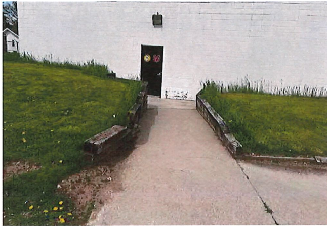
WOODEN RETAINER WALLS
