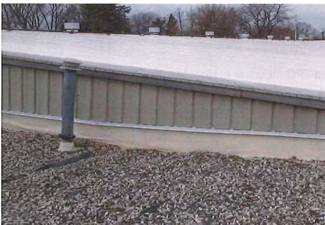
ARENA AND ICE PLANT ROOF
