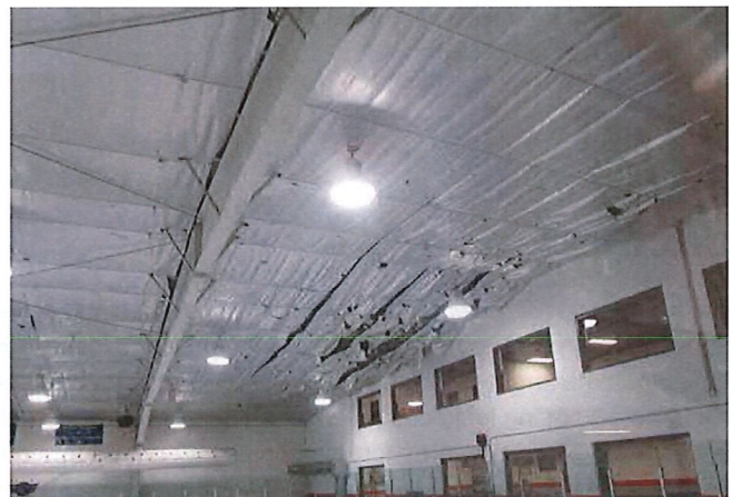
REFLECTIVE MEMBRANE RIPPED BY PUCKS
