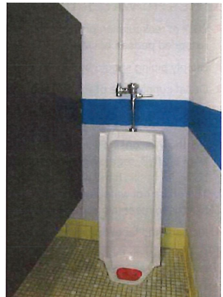
2ND LEVEL STALL URINAL MANUAL FLUSH
