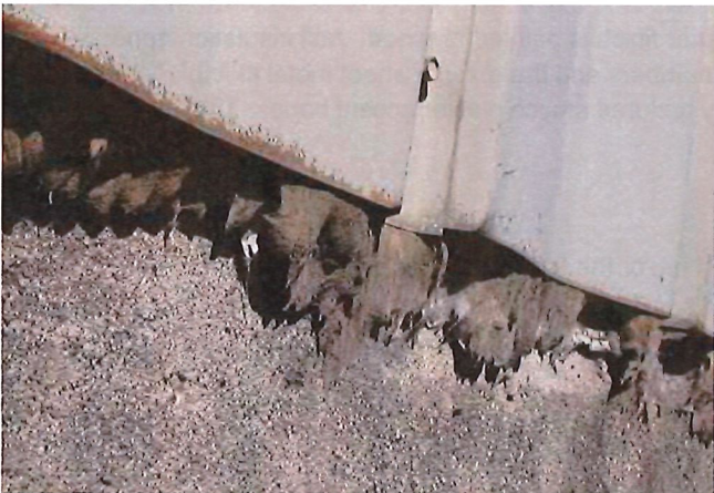
EXPOSED WALL INSULATION AT WALL BASE
