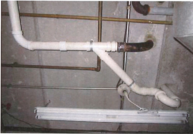
REPAIRS IN PVC
