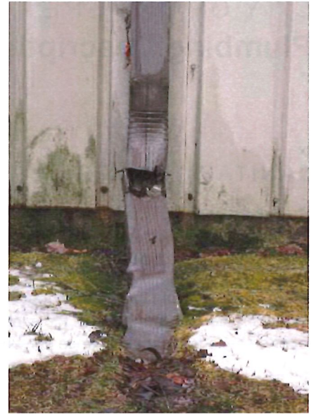
CRUSHED DOWNSPOUTS
