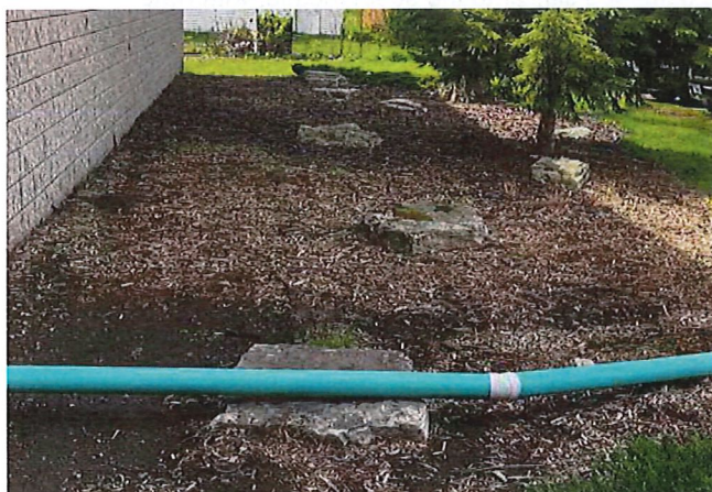
SURFACE ROOF DRAINAGE PIPE
