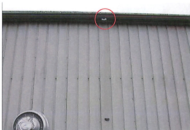
MISSING DOWNSPOUT
