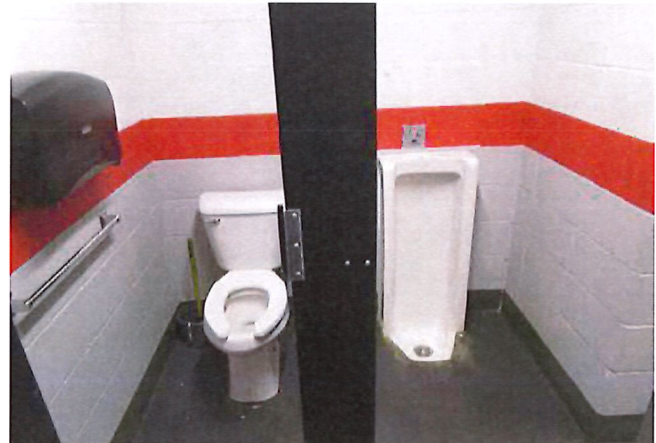
TYPICAL NON-ADA RESTROOM
