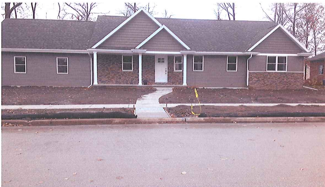
Terrace Walk at 2101 Ten Mile Drive
