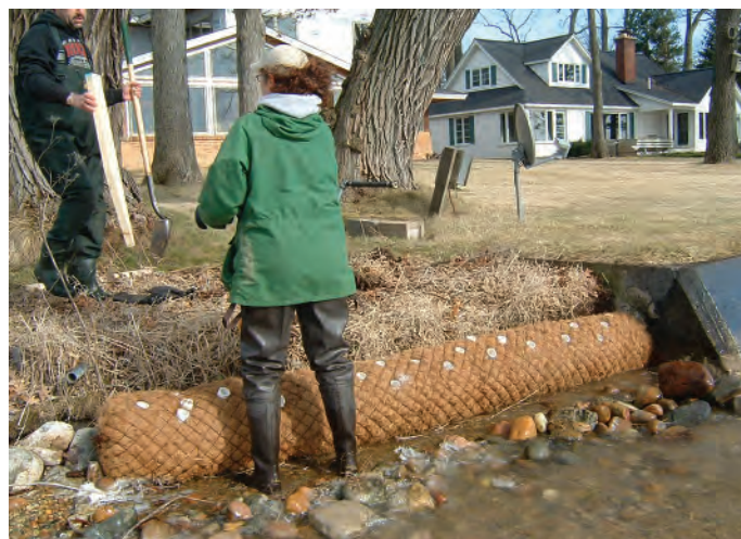
Figure 4.21. Coir log installation, March 2008. (Photo: Jane Herbert)
