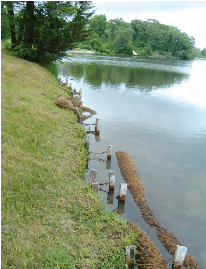
Figure 6.2. Poorly maintained coir logs can become a navigational hazard when displaced by wave action. (Photo: Jane Herbert.)
