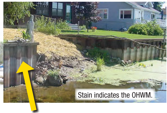
Figure 7.1. Arrows indicate common features used to estimate the ordinary high water mark on residential lakefront property. Common features may include changes in soils and vegetation and watermarks on seawalls.
