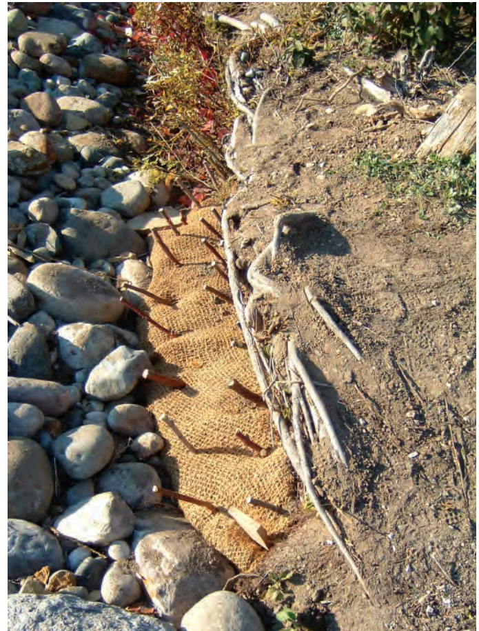
Figure 4.16. Autumn installation of dormant live stakes (foreground) and whips to repair shoreline damaged by an uprooted tree. (Photo: Jane Herbert.)
