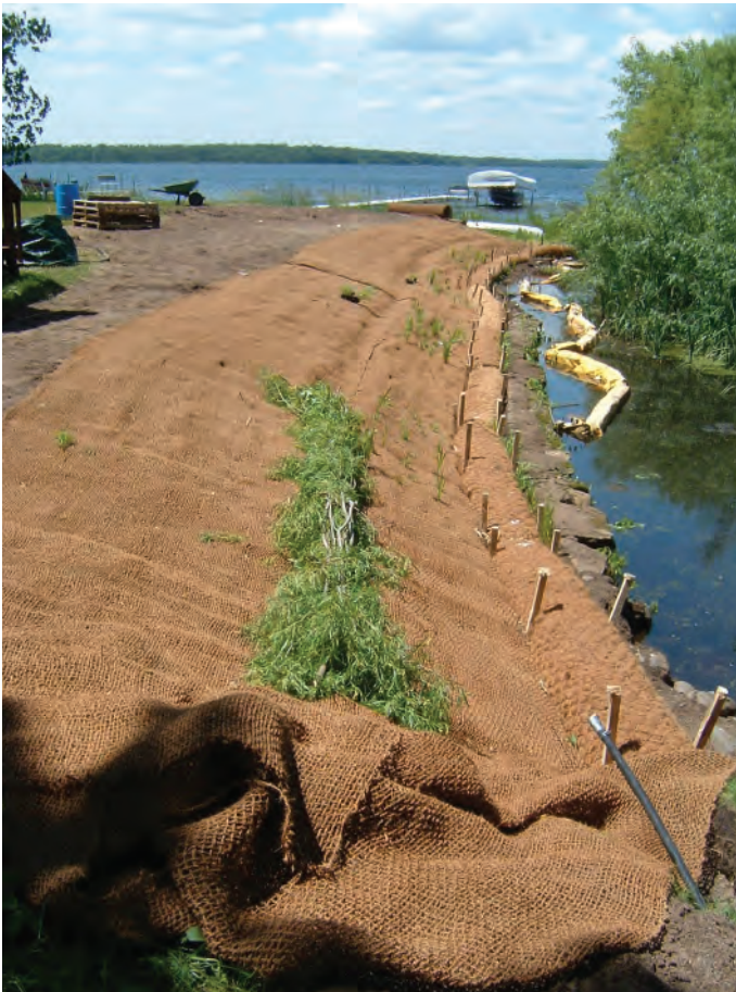
Figure 4.15. Wattles staked in to secure ECBs at their overlap. Notice how the upper blanket overlaps the lower blanket. (Photo: Jane Herbert.)
