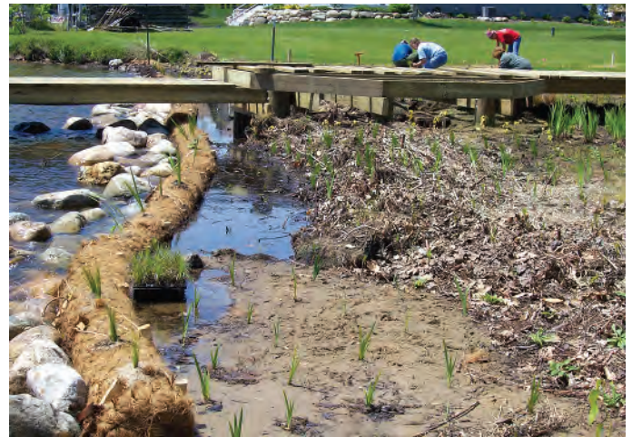
Figure 4.26. Planting native wetland plants in and behind the coir logs (May 2005). (Photo: JFNew.)
