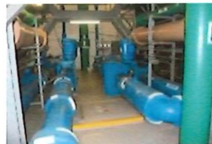
Pipe gallery painting
