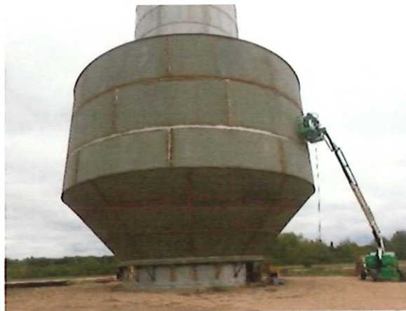
Wyoming, MN New Tank Construction 750,000 EWT
