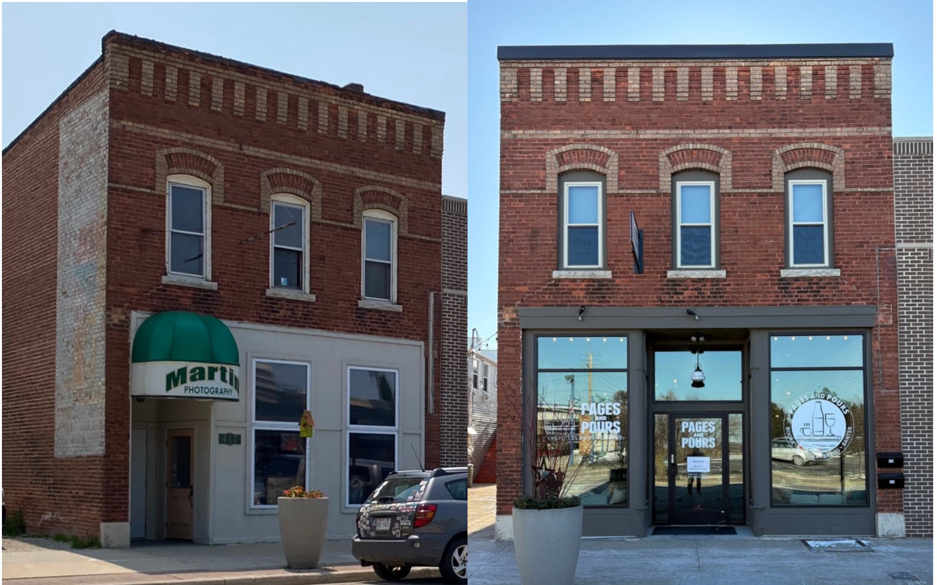
Above is the north façade of 415/417 Main with the before picture on the left and the after picture on the right. The new façade recreates the early 1900 design of the building with the large windows, showcasing the new bookstore and providing northern exposure natural light for the customers inside.
