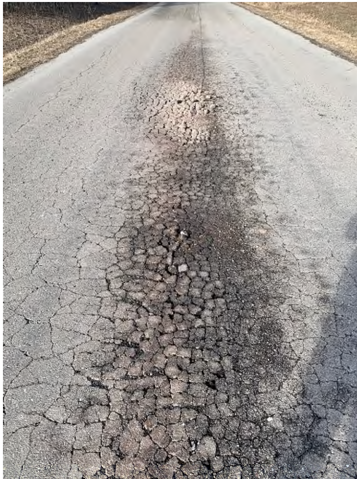
Figure 1 – Rockland Road looking west towards Old Plank Road
