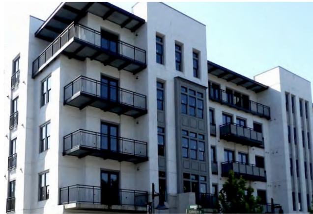
Figure 9-5. Examples of Balconies
