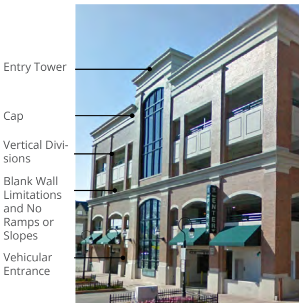
Figure 9-14. Illustration of Parking Structure
