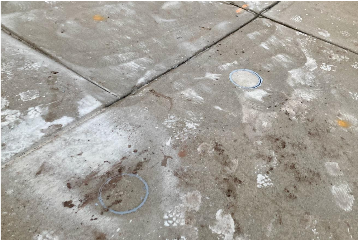
Figure 1 - Utility Coring at 1826 Saddlebrook Lane
