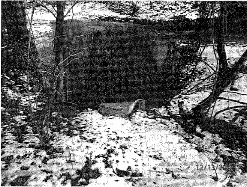
Downstream Side of Culvert – Viewing East
