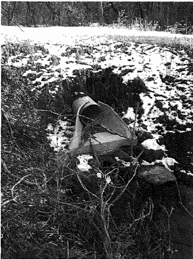
Upstream Side of Culvert - Viewing East - Note that two culverts stacked vertically.
