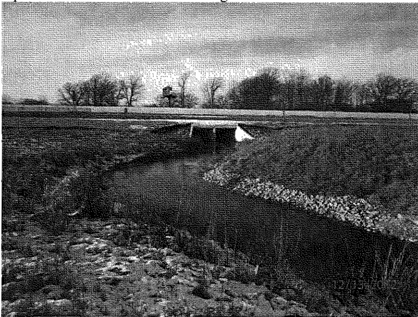
USH 41 Box Culvert – Upstream of City Culverts
