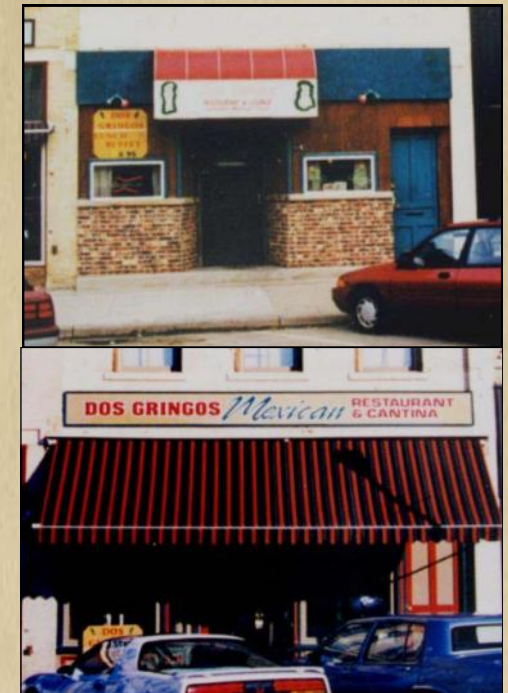
Recommended window replacement
