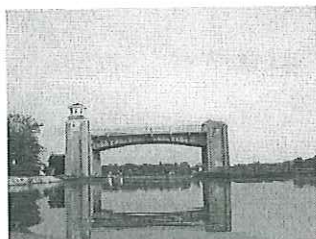
Looking south of retained bridge towers from Fox River Trail
