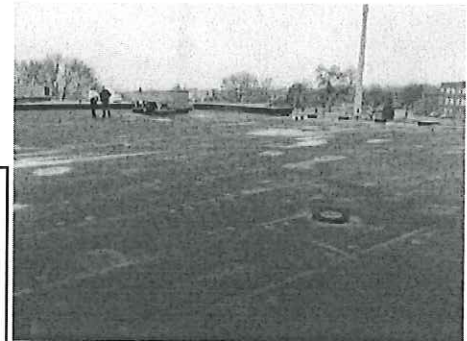
De Pere City Hall Current Green Roof Condition
