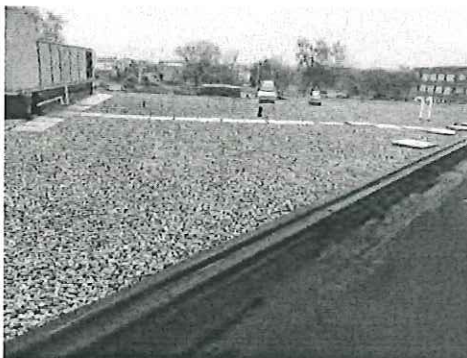
De Pere City Hall Current Green Roof Condition
