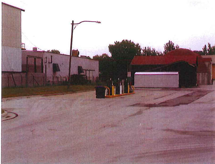
Fuel Island - Looking West
