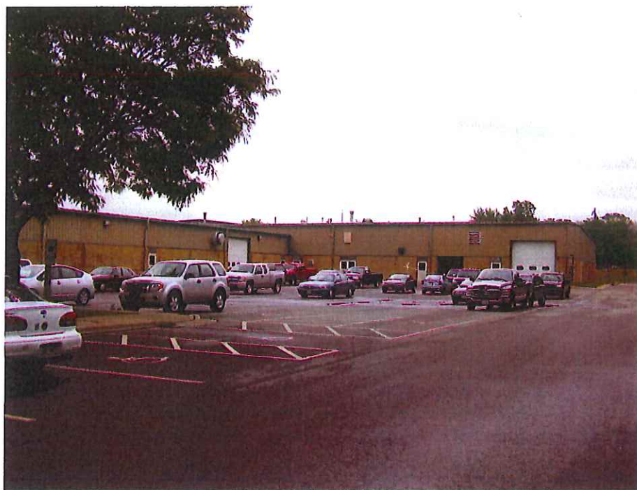
South side of facility/Employee Parking - Heated Garage (left) – Shops and Wash Bay (Right)
