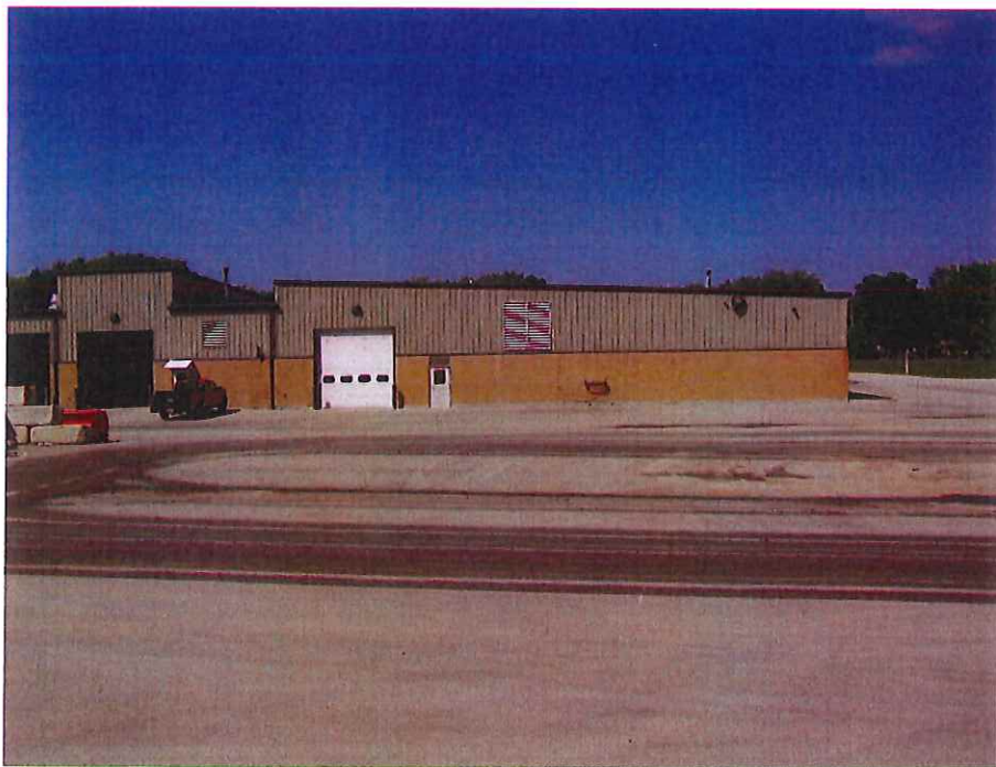
Westside – Heated Parking
