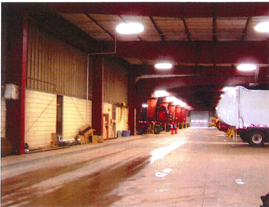
Existing Vehicle Aisle (Vehicles projecting into Vehicle Aisle – Safety Cones)
