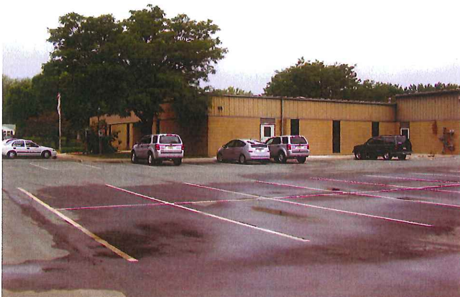
Administrative Offices/Employee Support
