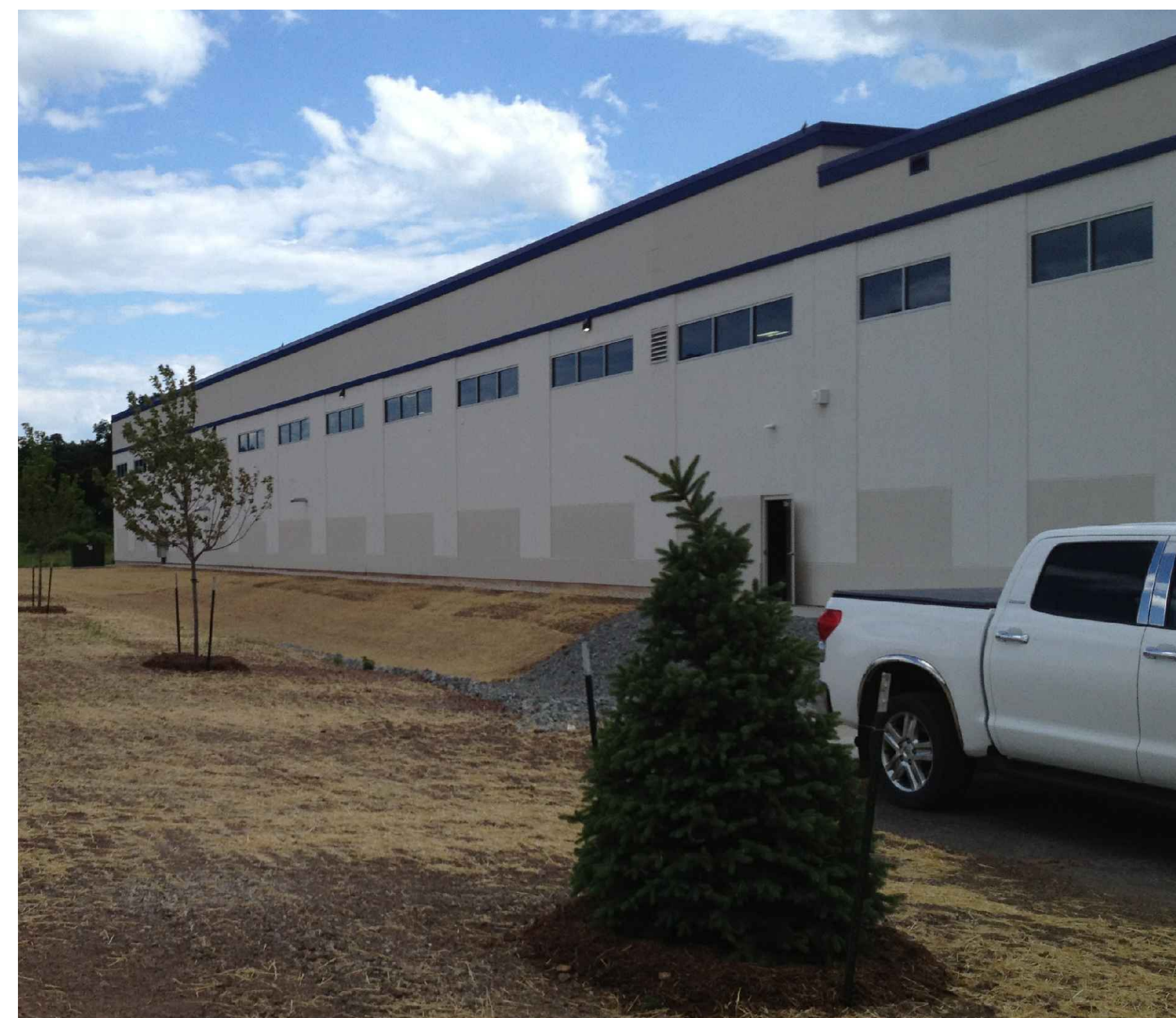
3 A3.1 EXISTING EXTERIOR PHOTO NOT TO SCALE
