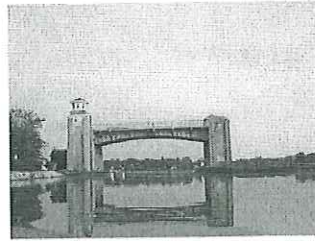
Looking east of retained bridge towers from Fox River Trail
