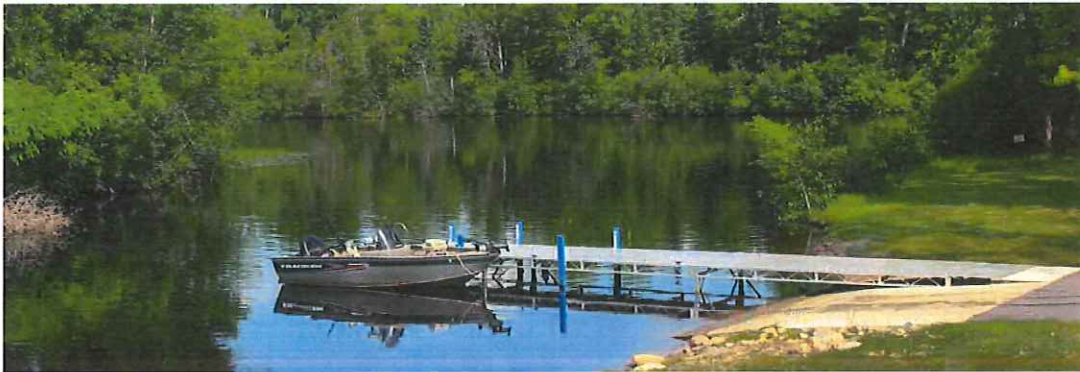
Boyce Drive Boat Landing | City of Rhinelander Improvements to the Boyce Drive Boat Landing include a new boat ramp, new ADA-accessible dock, new ADA-compliant restroom facility, and parking.
