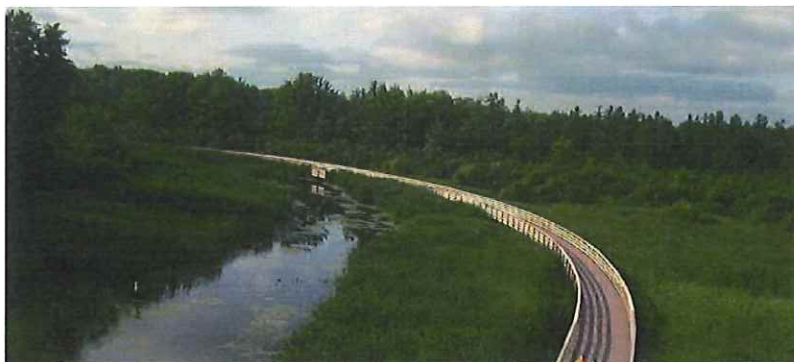
Spring Brook Trail | City of Antigo This two-mile trail connects the City's downtown, an elementary school, and one of the community's parks. Our team developed a project schedule and design that allowed for winter construction to avoid impacting the wetland the trail spans. The boardwalk is made of treated lumber with recycled polyethylene decking.
