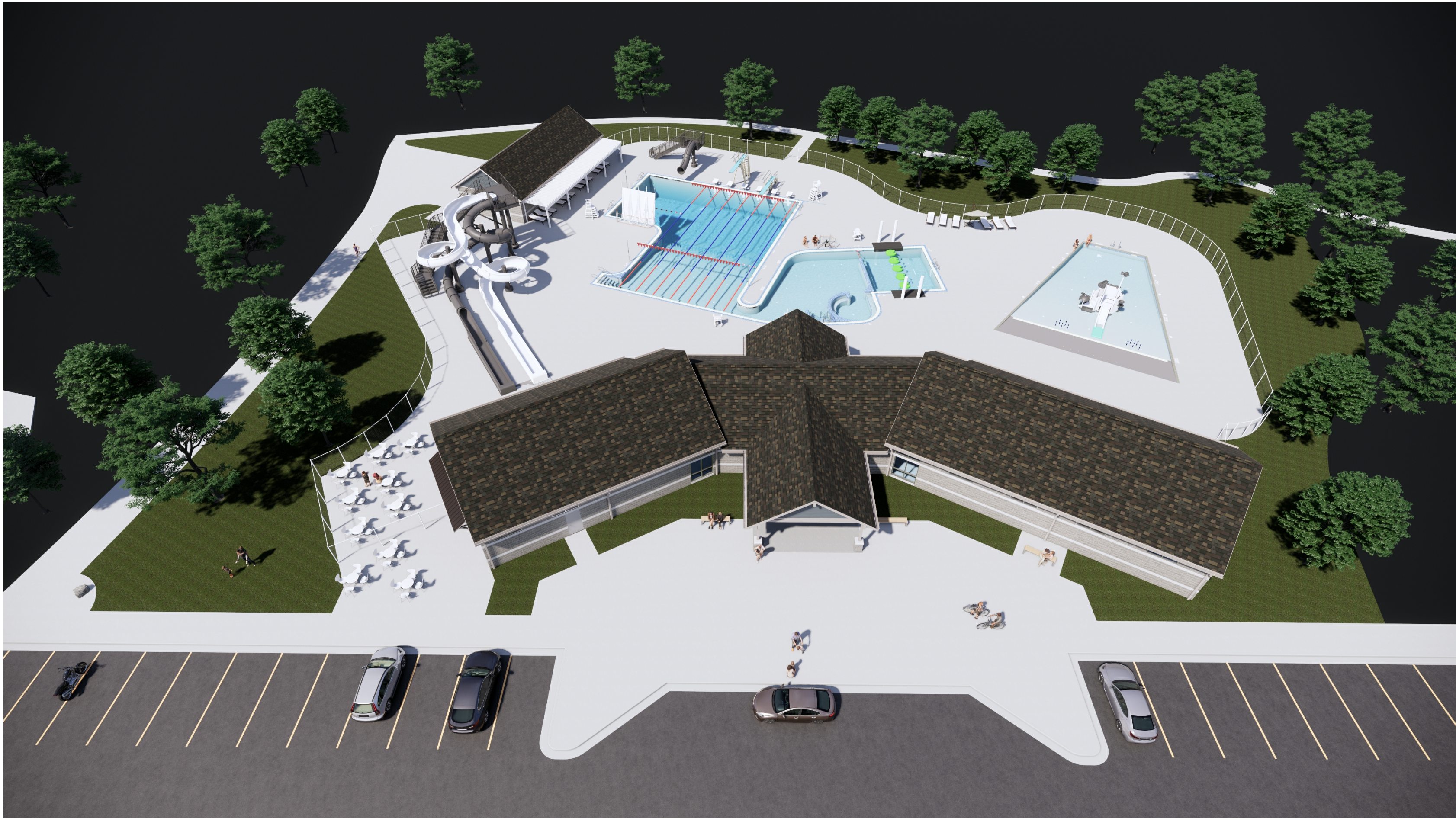
AERIAL VIEW - LOOKING NORTH
