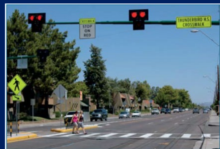
A Pedestrian Hybrid Beacon (PHB) in Phoenix, Arizona provides protection for pedestrians near a high school.
