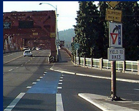
Above and Below: Colored sections of bicycle lanes typically delineate the areas of conflict where vehicular traffic and bicycle traffic will cross paths.
