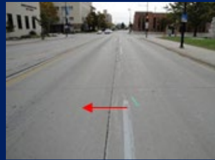
Below: Multi-lane street striping.
