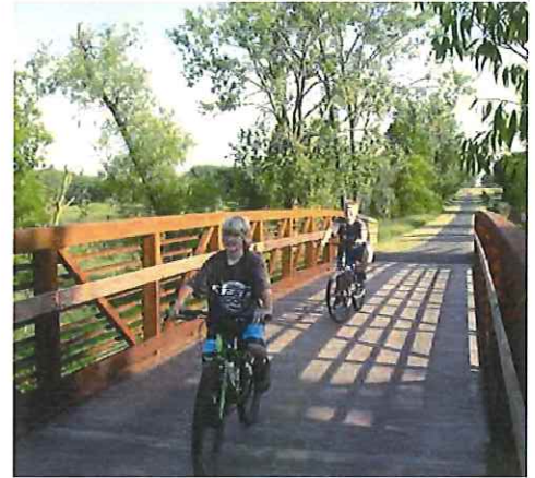
MSA worked with Ramsey County staff to provide wetland delineation, surveying, design, permitting, and construction related services for the extension of Rice Creek Trail in Maplewood, MN.
