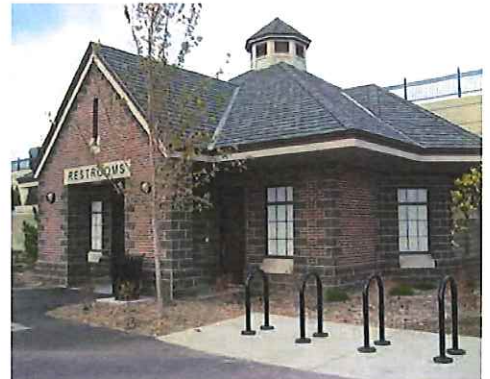
MSA's architects designed this new public restroom facility located in Canal Park along the Lake Superior shoreline walking path.
