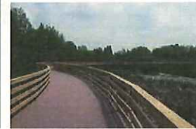
Spring Brook Trail | City of Antigo This two-mile trail connects the City's downtown, an elementary school, and one of the community's parks. Our team developed a project schedule and design that allowed for winter construction to avoid impacting the wetland the trail spans. The boardwalk is made of treated lumber with recycled polyethylene decking.
