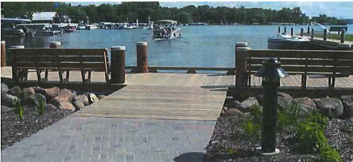
Deacon Mills Park Wharf | City of Green Lake MSA provided design services for the seawall replacement, new wharf construction, pedestrian boardwalk, adjacent brick paver walkway, and landscape improvements.
