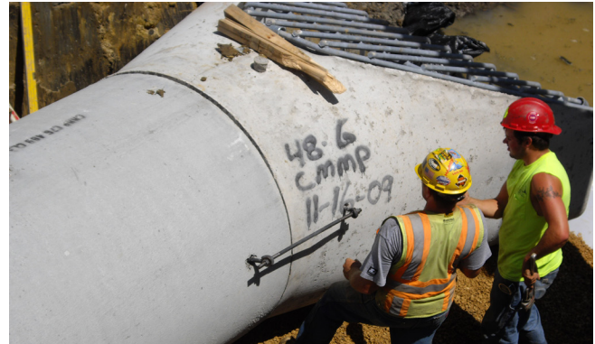
REEDSBURG, WI, FLOOD RECOVERY & MITIGATION
