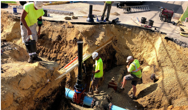
DODGEVILLE, WI, SPRING STREET RECONSTRUCTION
