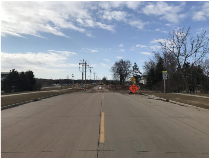
Area where power poles would be buried
