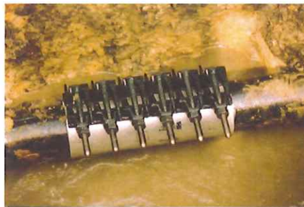
Leak repaired.
