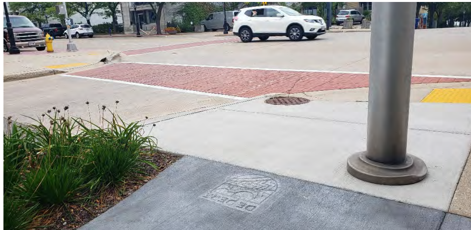
Figure 1: Brick-paved Crosswalks Near Walsh Plaza.
