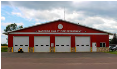
Marengo Fire Hall
