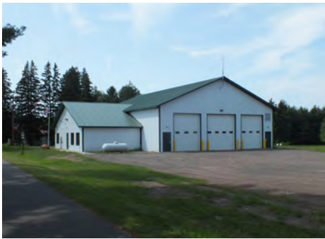
Port Wing Fire Hall
