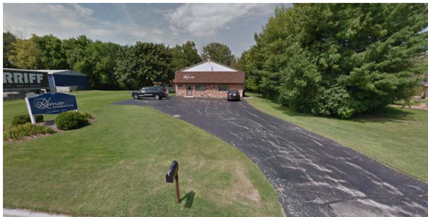
Figure 2: Existing Building – Former Kimco Engraving
