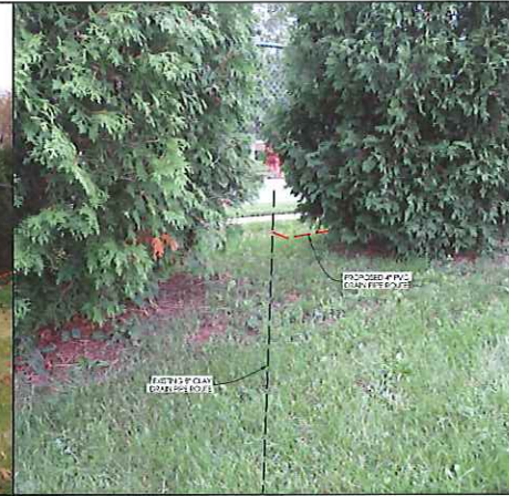
EXISTING OVERFLOW DRAIN FROM TOWER BASE
