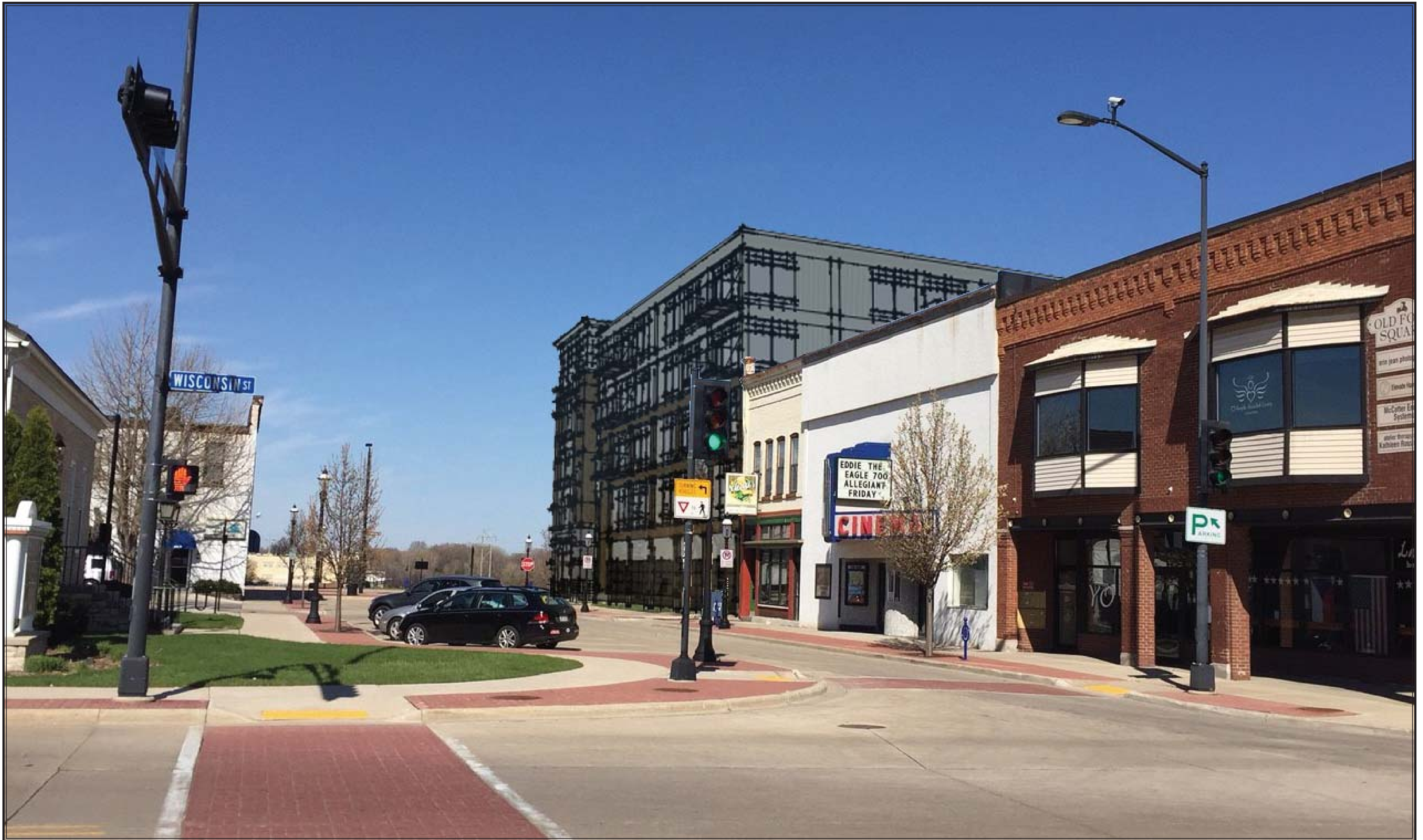
Contextual View from George Street
