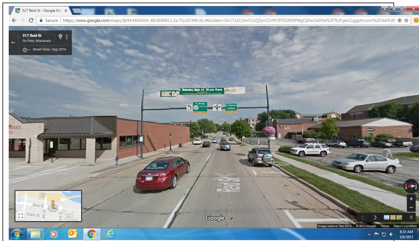
Overhead Street pole
