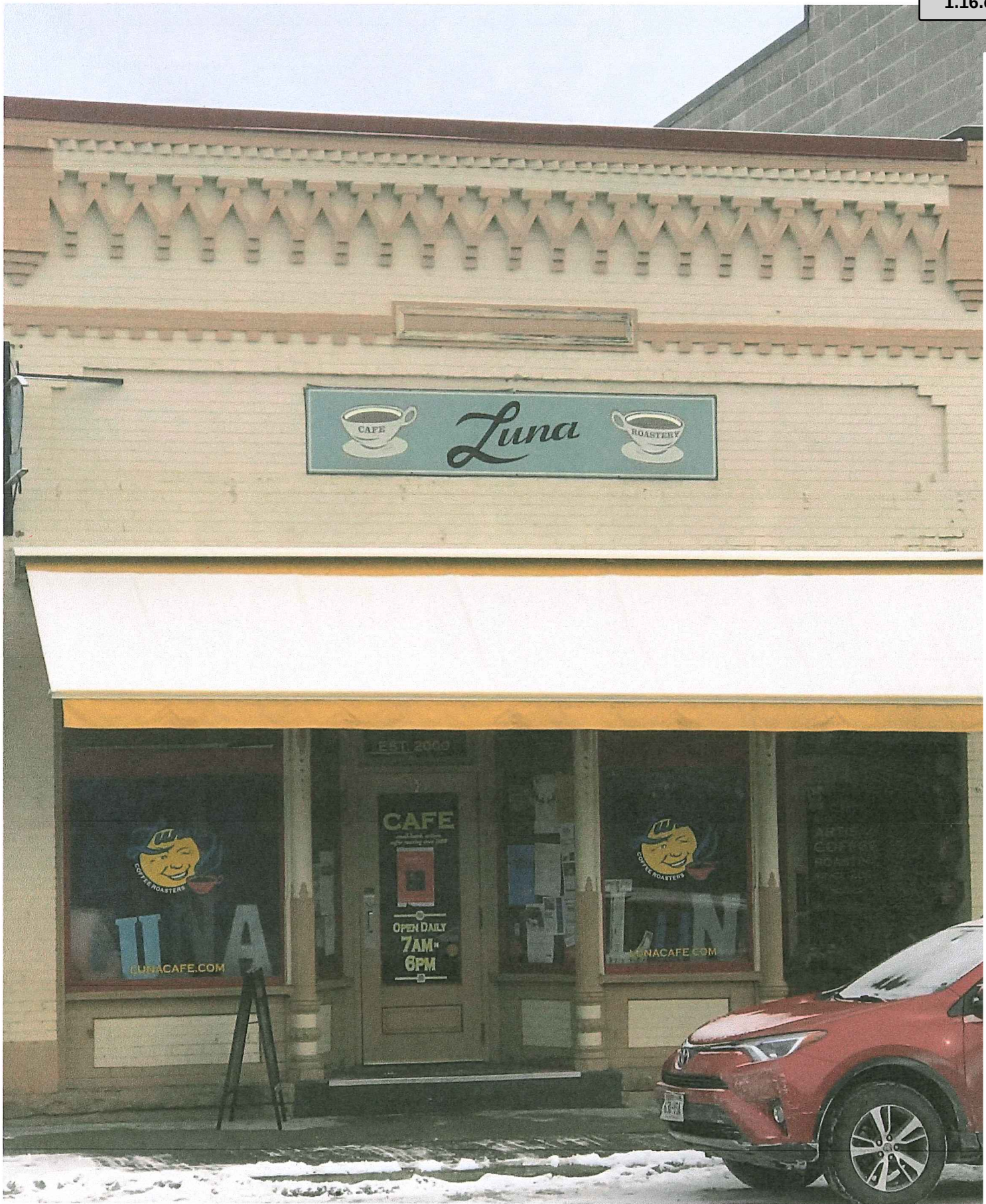
Attachment: Exhibit A (Supplement) Luna Facade Grant Quotes 5-2018 (6928 : Reso #18-48 Approving Facade Improvement Project and
