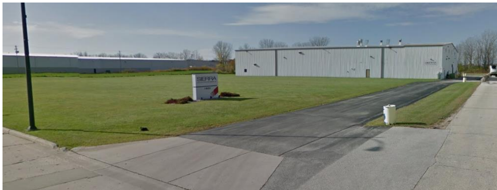
Figure 2: Existing Building – Former Kimco Engraving
