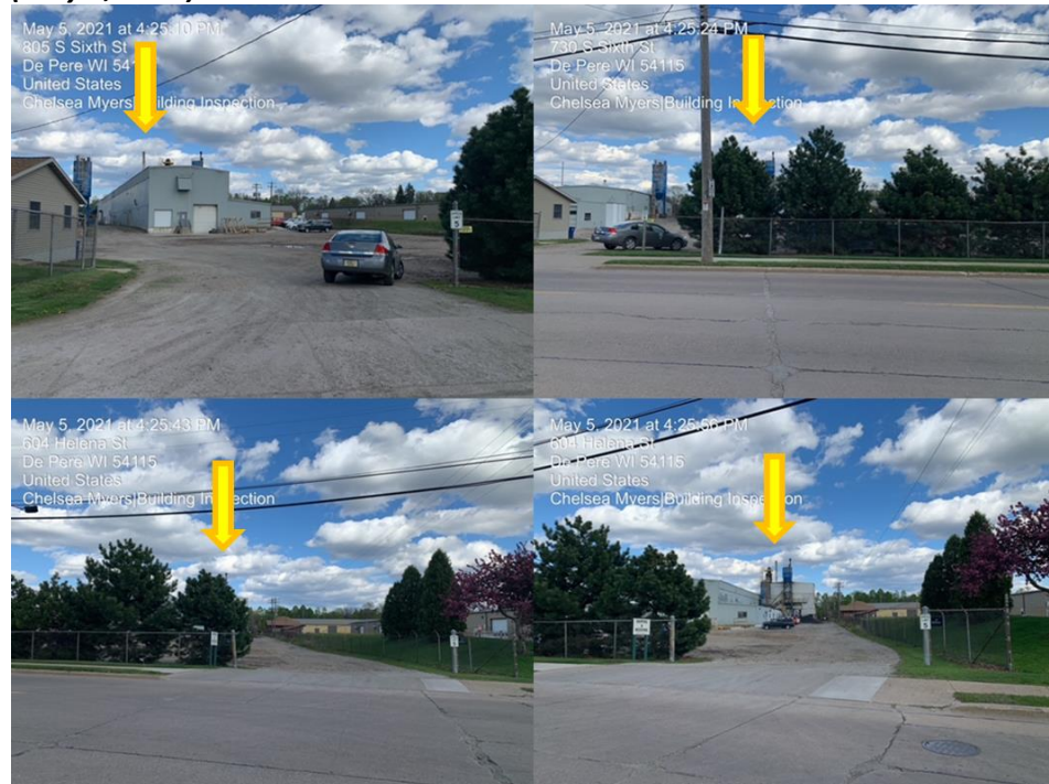
View of existing exhaust stack from middle and south driveways on Sixth ST (May 5, 2021):
