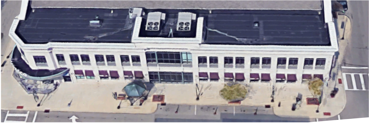
Figure 3-33. Rooftop Utilities Screened from the Public Way by a Parapet
