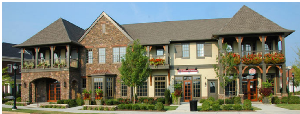
Figure 3-3. Illustrative Examples of Commercial Manor Building
