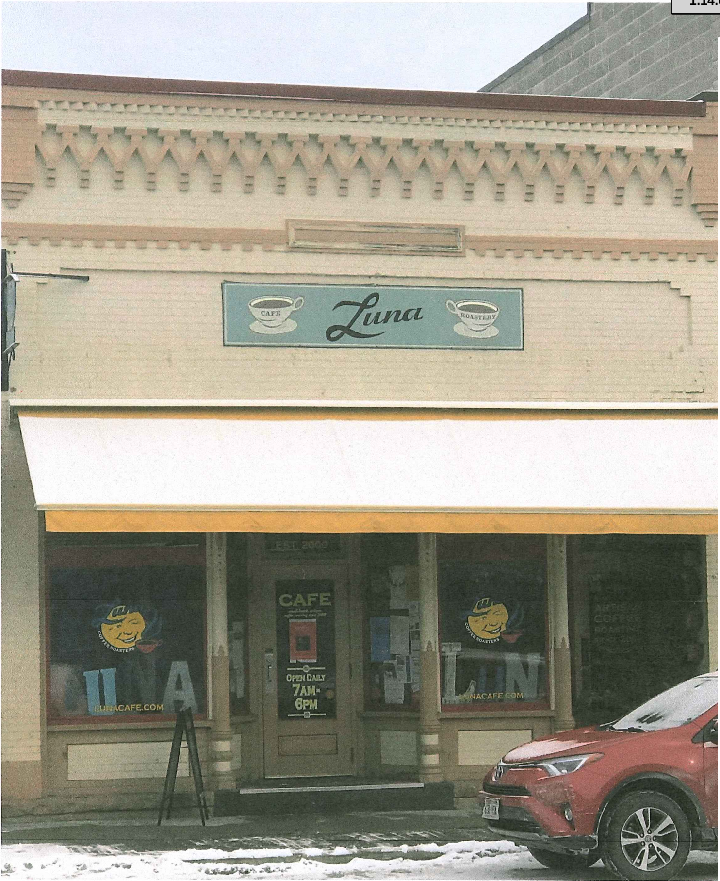
Attachment: Exhibit A (Supplement) Luna Facade Grant Quotes 5-2018 (7026 : Reso #18-48 Approving Facade Improvement Project and
