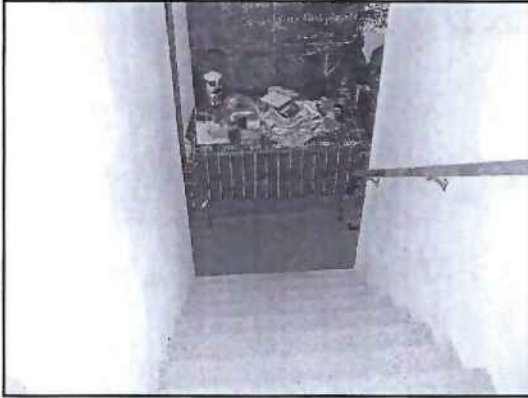
Stairs to basement area
