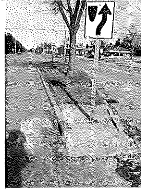
Looking North from the South end of the median in Webster Avenue
