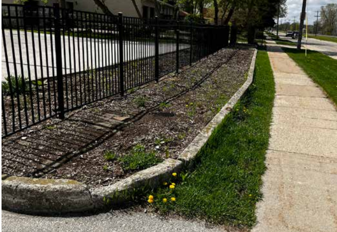
RETAINING CURB AT FORT HOWARD DRIVE
