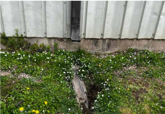
DOWNSPOUT WASHOUT
