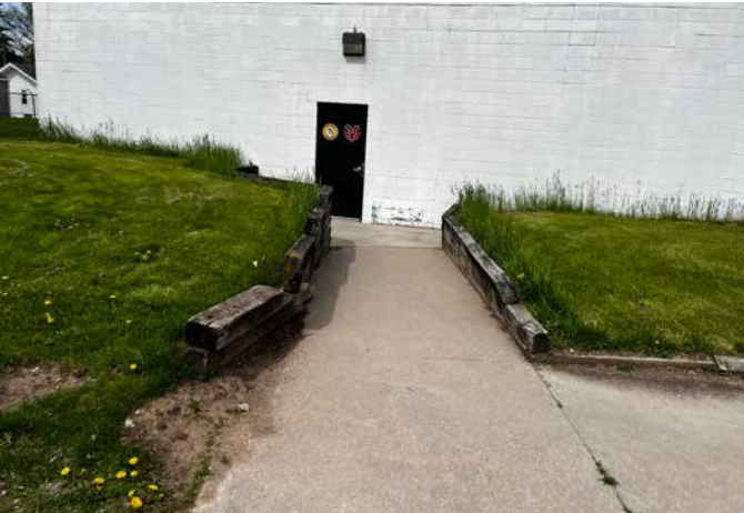
WOODEN RETAINER WALLS
