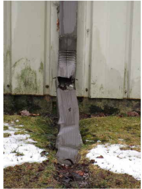
CRUSHED DOWNSPOUTS
