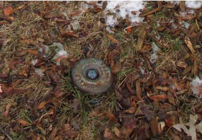
WATER SERVICE SHUT-OFF VALVE
