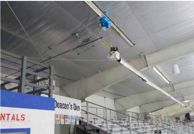
INFRARED HEATERS
