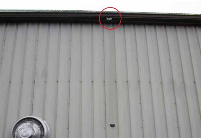
MISSING DOWNSPOUT
