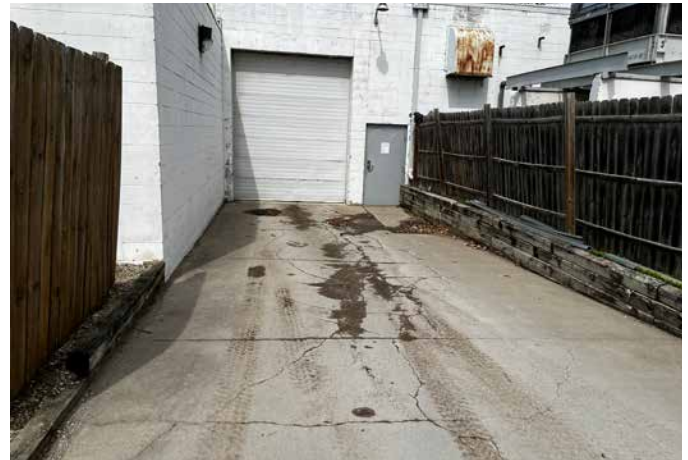
ZAMBONI ACCESS DOOR
