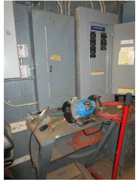
WORK BENCH CONFLICTS WITH WORKING SPACE OF BRANCH PANEL
