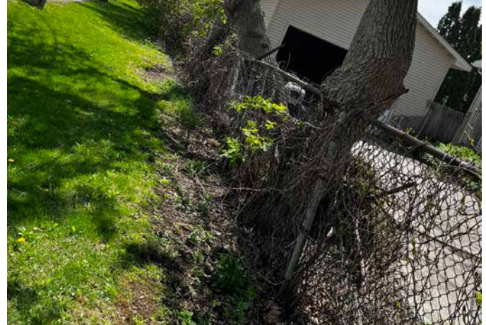
OVERGROWN TREES AT SOUTH PROPERTY LINE
