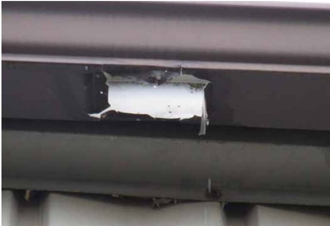
MISSING DOWNSPOUT
