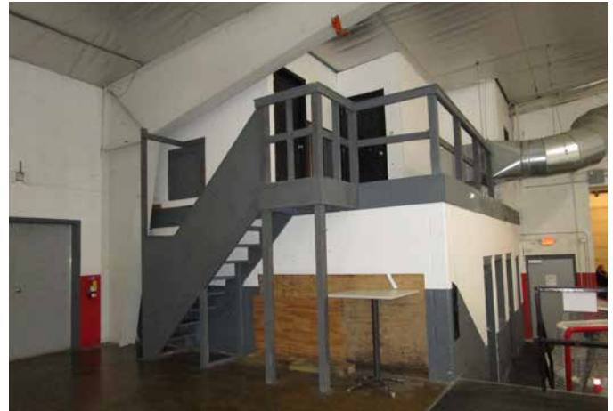
WOODEN STAIRS TO DEHUMIDIFIER EQUIPMENT
