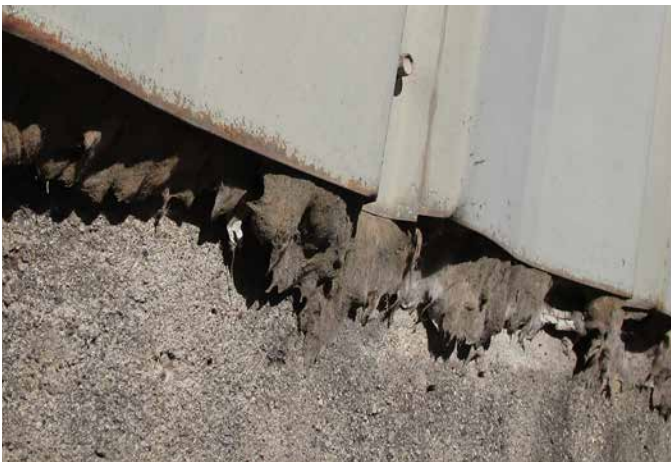
EXPOSED WALL INSULATION AT WALL BASE
