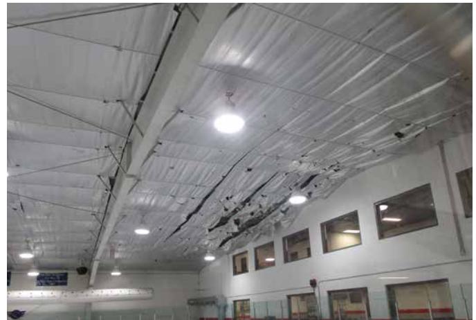
REFLECTIVE MEMBRANE RIPPED BY PUCKS
