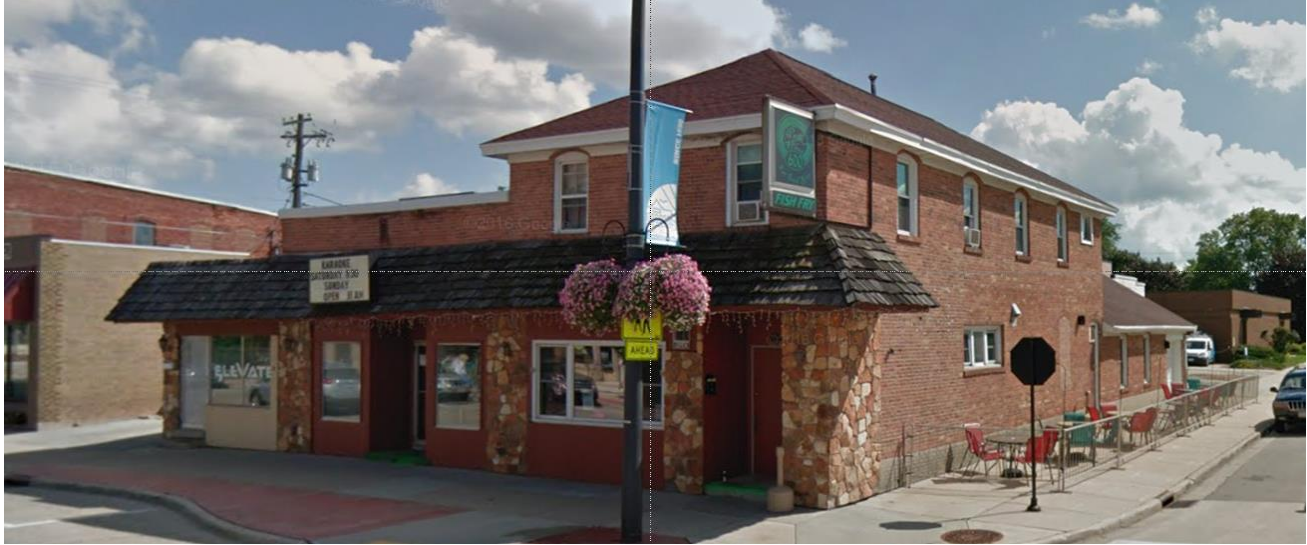
Existing Front Facade
