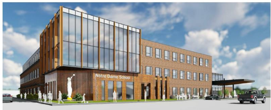
Street view northwest corner (Superior & George St)
