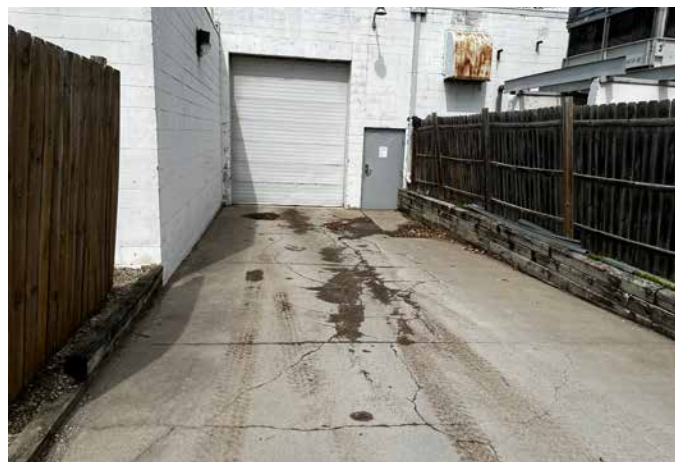
ZAMBONI ACCESS DOOR
