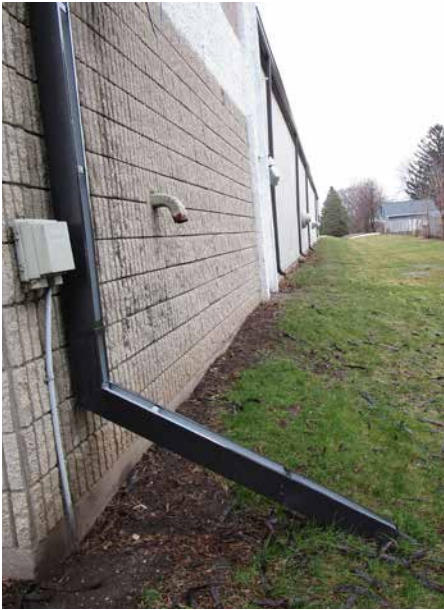
GUTTER AND DOWNSPOUTS
