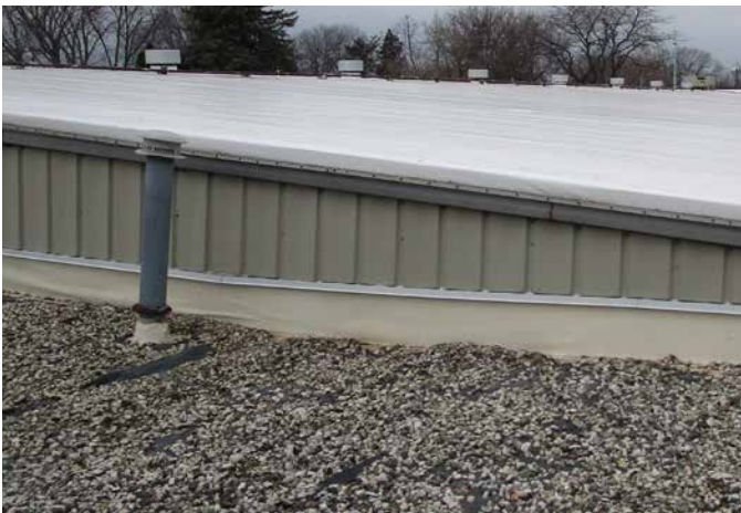
ARENA AND ICE PLANT ROOF
