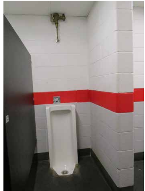
STALL TYPE URINALS W/SENSOR OPERATED FLUSH
