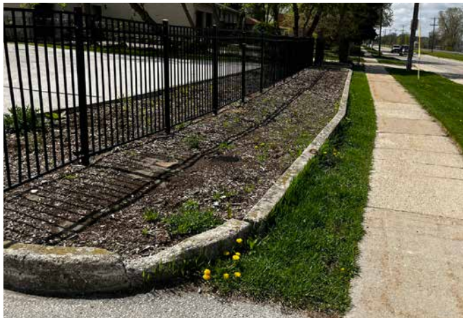
RETAINING CURB AT FORT HOWARD DRIVE
