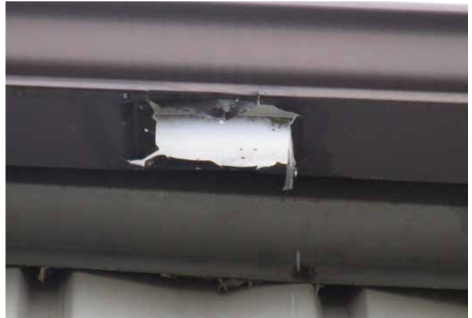
MISSING DOWNSPOUT
