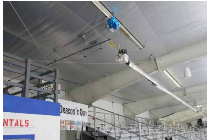
INFRARED HEATERS
