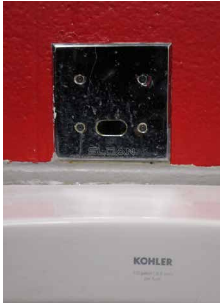
URINAL SENSOR OPERATED FLUSH
