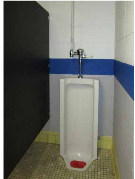
2ND LEVEL STALL URINAL MANUAL FLUSH
