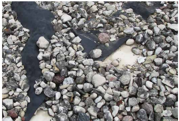
ICE PLANT ROOF
