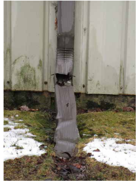
CRUSHED DOWNSPOUTS
