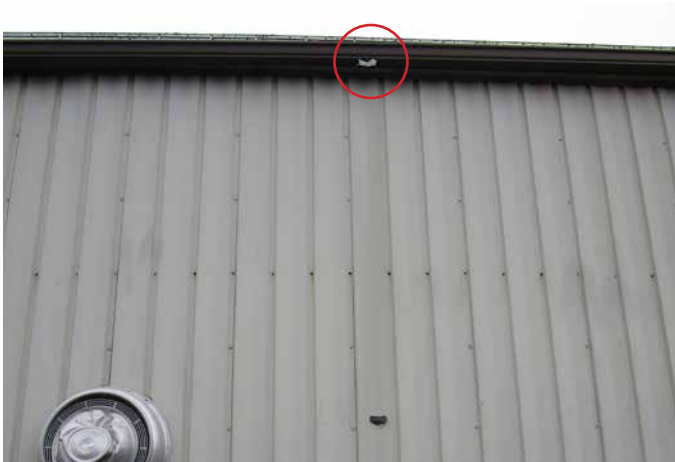
MISSING DOWNSPOUT
