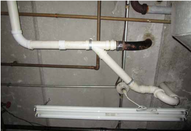
REPAIRS IN PVC
