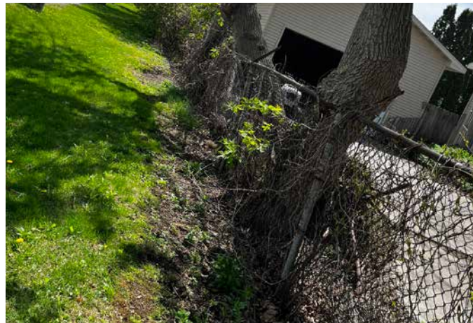
OVERGROWN TREES AT SOUTH PROPERTY LINE
