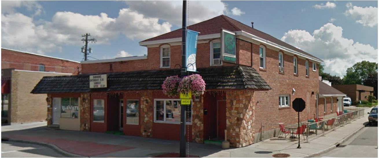
Existing Front Facade
